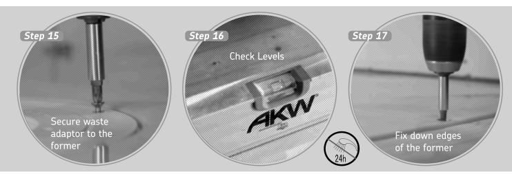
**Step 17. Fix down** – only when the former is fully supported and level with the surrounding floor, apply an adhesive or mastic to all supporting surfaces and screw down the edges of the former onto the joists and noggins. Foam should not be used as a load bearing support as it will break down under repeated product use. Do not overtighten the screws.
